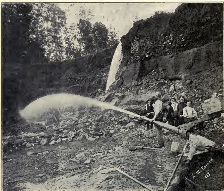
Hydraulic mining on the Klamath River.
